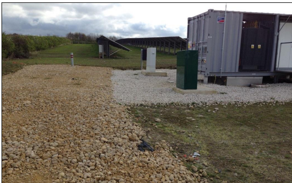
Plate 14: Typical Type 2 Aggregate at Solar Farm 34
